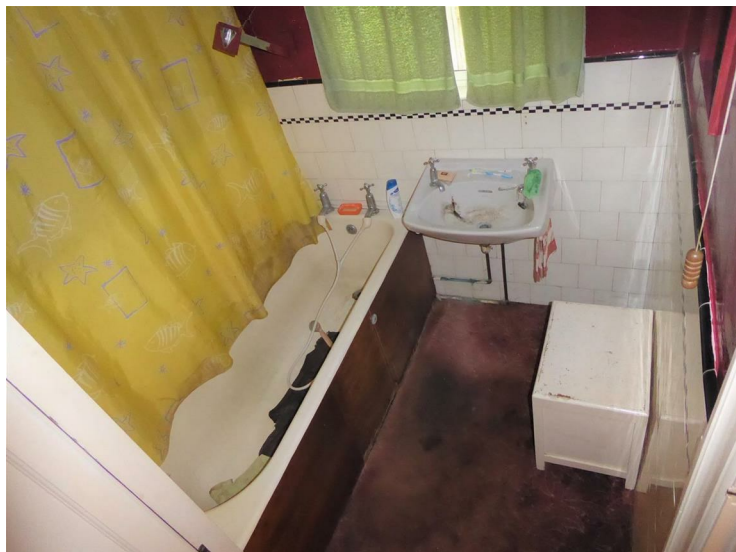
Panel enclosed bath, wash hand basin, part tiled walls, side aspect secondary glazed window, airing cupboard housing cylinder tank.
